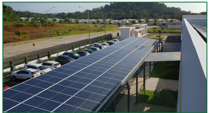
Solar power panels installed on carports at SABIS® Costa Verde
