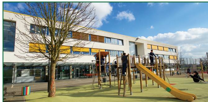
ISF International School Frankfurt Rhein - Main, Germany
